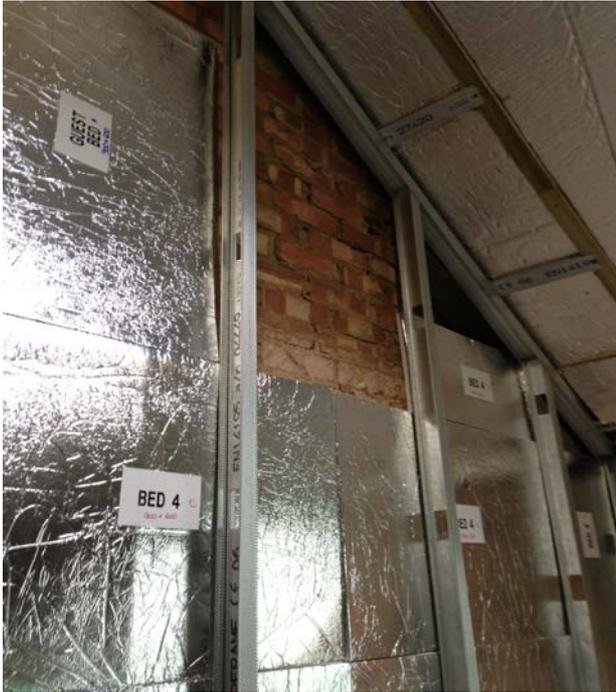
The exact wall build-up was as follows - Existing wall / 15mm VIP with 10mm EPS backing / 60mm Gyproc stud / 12mm Plywood boarding / 12.5mm Plasterboard / 3mm skim coat.
