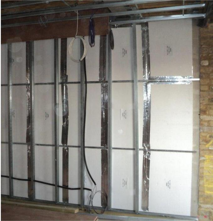
In order to overcome this issue Studio Indigo designed a system which created an 87mm clearance between the VIPs and the internal face of the wall. This clearance would allow for internal fixings at a later date without the fear of puncturing the panels.
